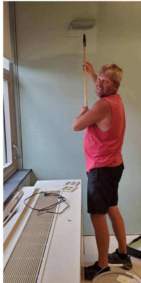
John Haskins puts a fresh coat of paint on the technology office walls at W.T. Hoag.
